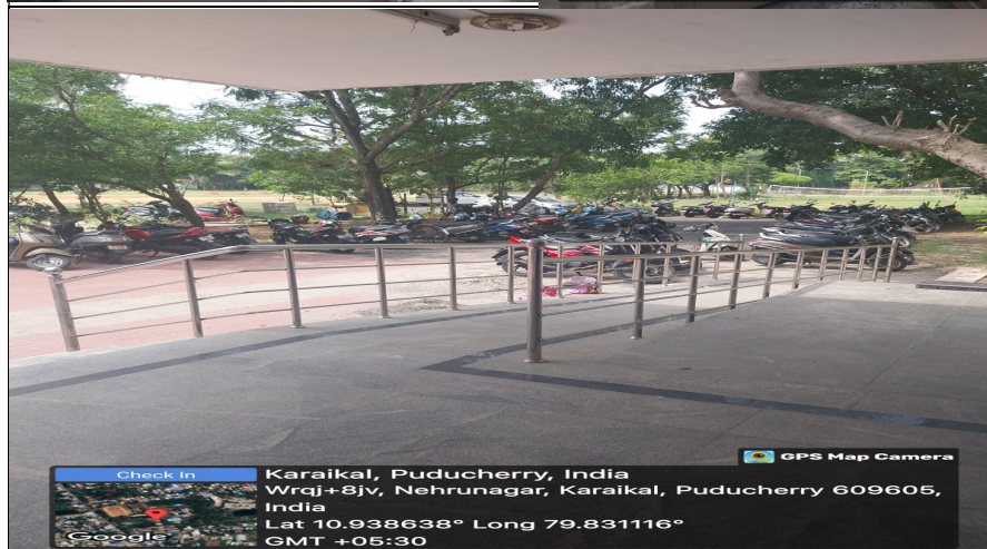
Wheelchair Ramp for Differently abled Persons
